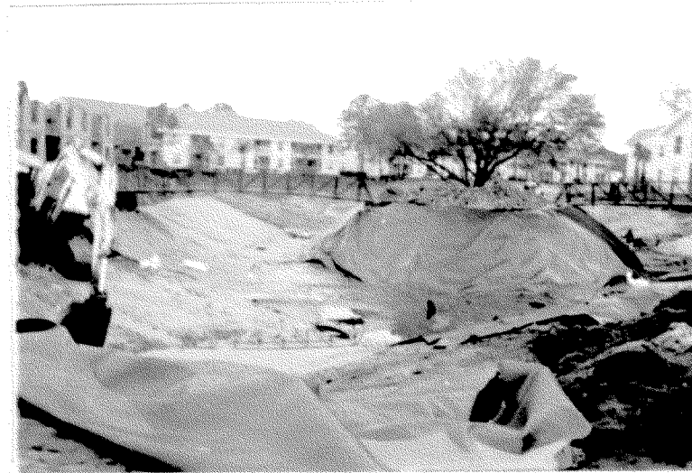
Fig. 9 Installation of geomembrane on island slope
