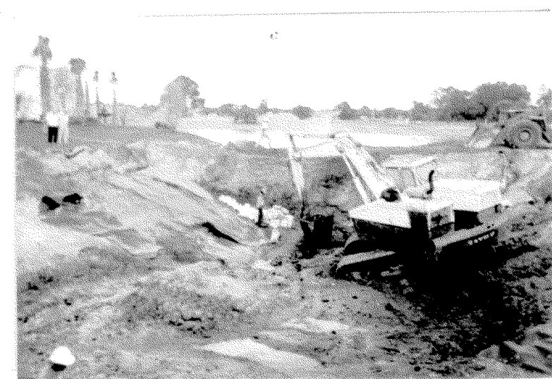
Fig. 6 Damming lake into halves and bottom grading (note rear portion of lake full with water)
