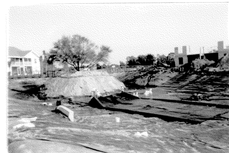
Fig. 8 Preparation of island slope with geotextile
