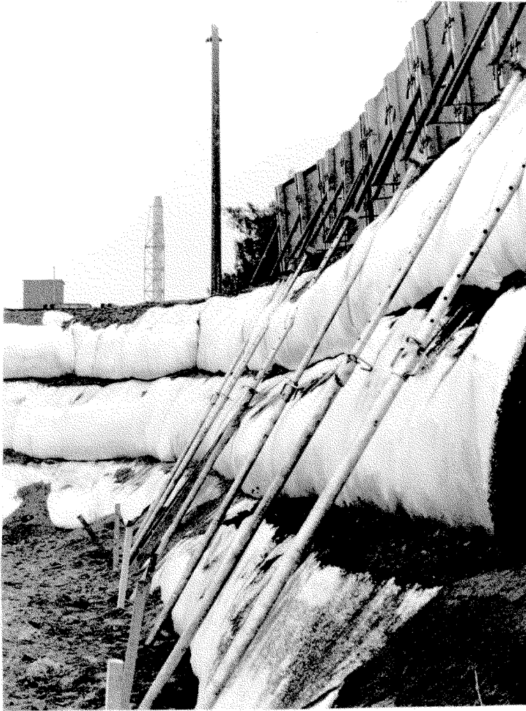
Fig.2 View of dam under construction
