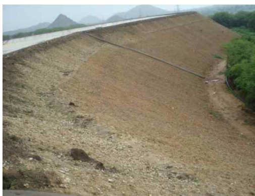
Figure 5. Pictorial view of outer slope before turfing
