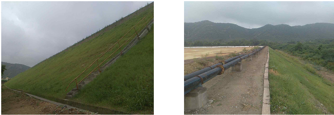
Figure 6. Outer slope after erosion control
