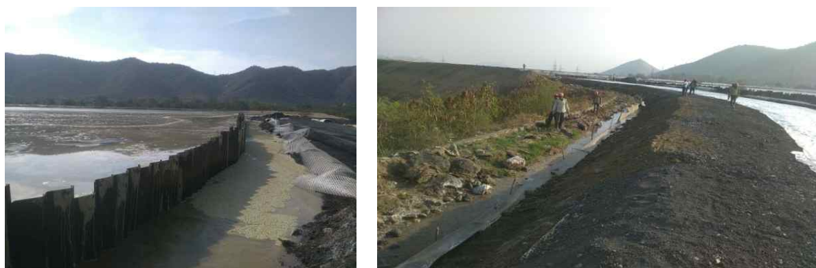
Figure 9. Construction of embankment on geocell strengthened inner base & sheet piling
