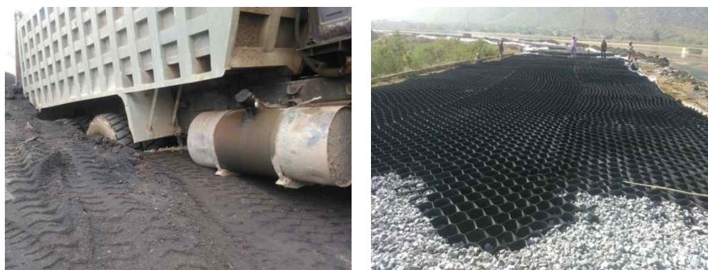
(a) (b) Figure 8. Application of geocells for strengthening of inner base
