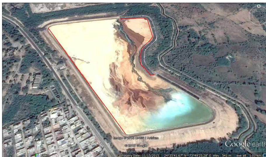
Figure 1. Overall view of the landfill site
