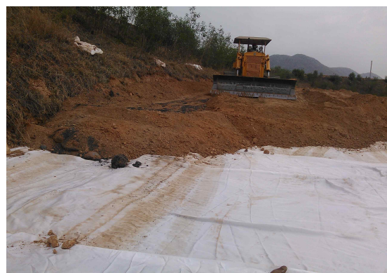
Geotextile (High strength) reinforcement at intervals
