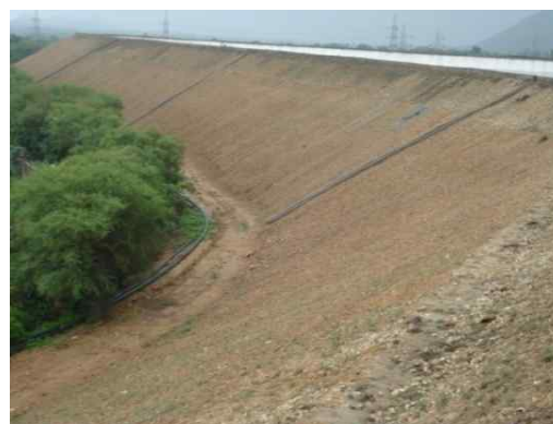
Figure 5. Pictorial view of outer slope before turfing
