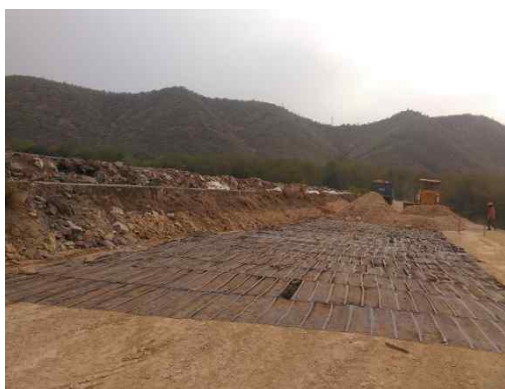
Geogrid reinforcement at base/intersection
