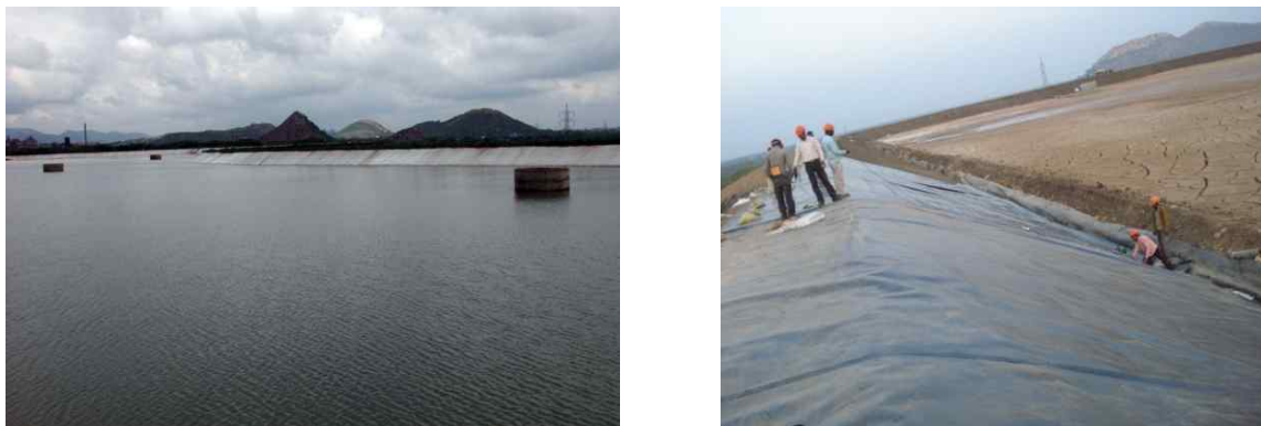
Figure 11. HDPE liner covered with geotextile protection layer
