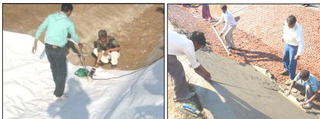
Photographs 6 and 7. Restoration of Tanchha Distributary
