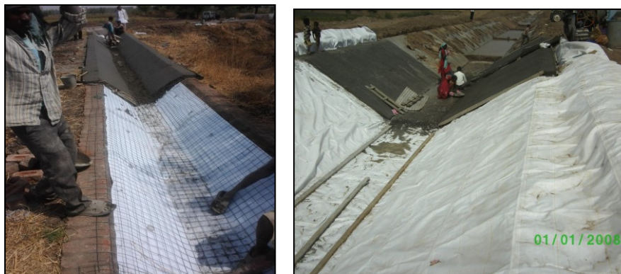
Photographs 8 and 9. Restoration of Keshlu minor and Vadodara Branch Canal
