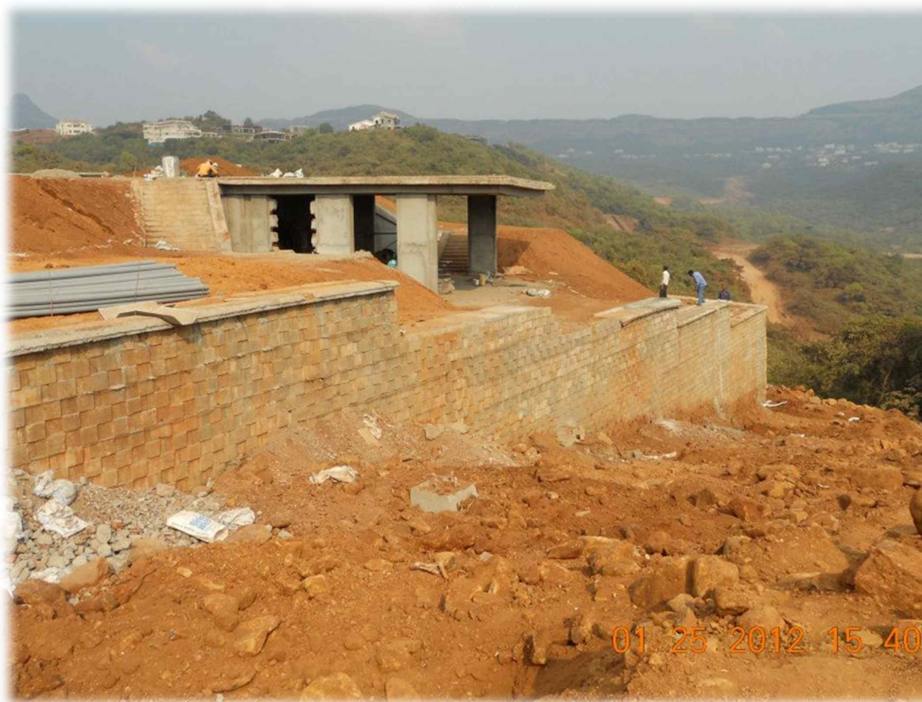
Figure 5. Photographs during execution of RS block wall
