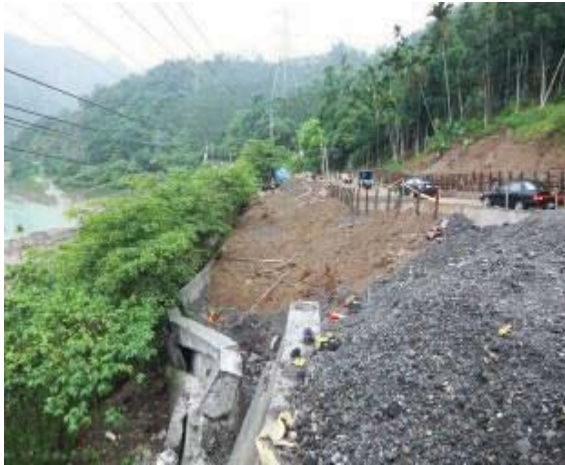
Fig. 2 Temporary solution for upper slope
