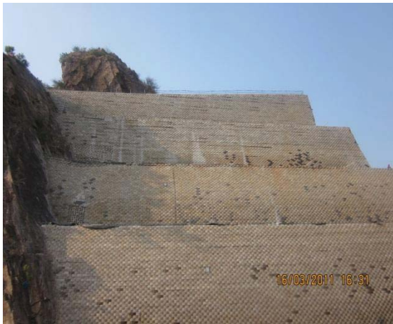
Fig. 9 A view of the completed tiered reinforced soil wall at location-1
