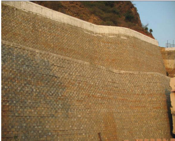
Fig. 8 A view of the completed tiered reinforced soil wall at location-1
