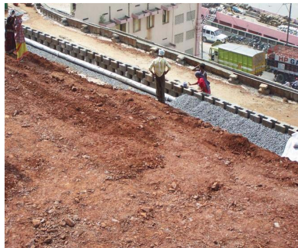
Fig. 7(b) Aerial views of fascia drainage system
