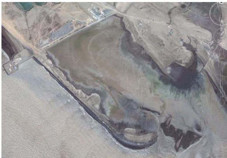
Fig. 7 Areal view of the port backup facility after land reclamation using geo-system as core material
