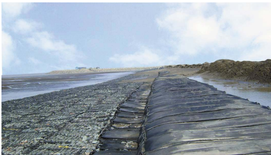
Fig. 9 Arrangement of geotextile containers and PP rope gabions in progress
