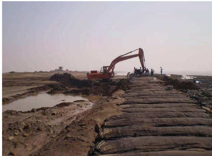
Fig. 5 During filling of the geotextile containers with local available material
