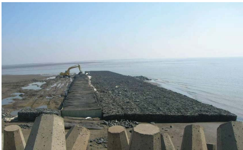
Fig. 3 During construction of apron and geotextile containers
