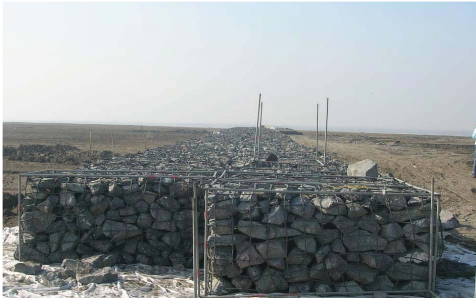
Fig. 4 During filling of PP rope gabion using steel frames
