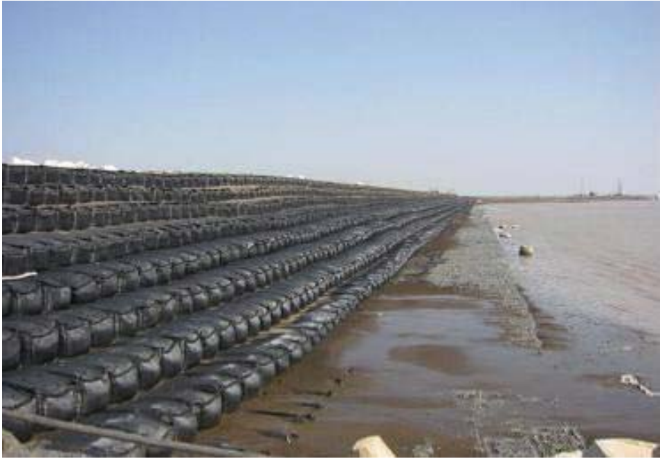
Fig. 10 Final arrangement of geotextile containers shore protection system
