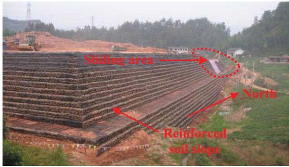
Fig. 2 Panoramic view of the reinforced soil slope.
