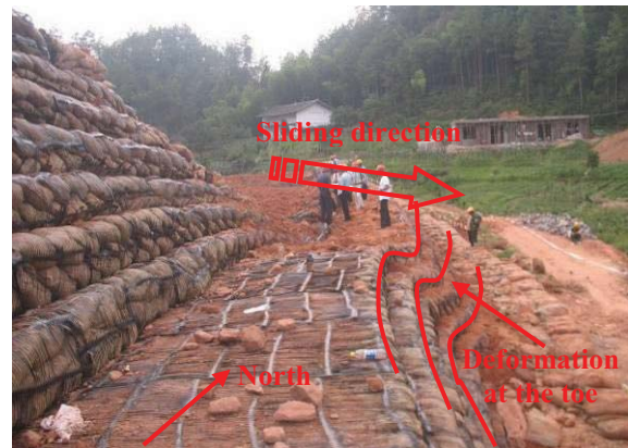
Fig. 9 Failure sketch of the reinforced soil slope.
