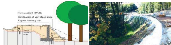
Fig. 5 Road construction alternatives at Gänsbergspange Idstein, Germany
