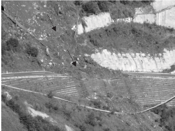
Fig. 6 Detail: road after landslide.
