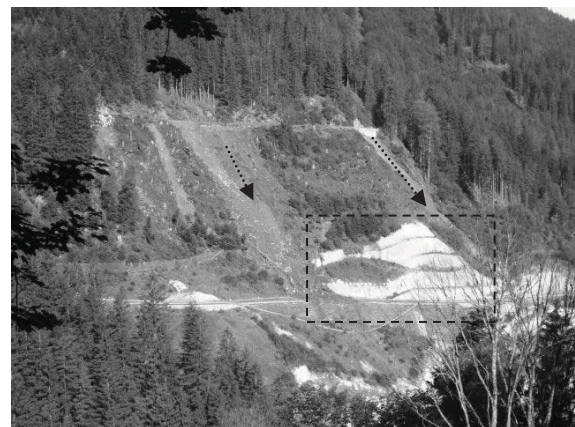
Fig. 5 Road after landslide.
