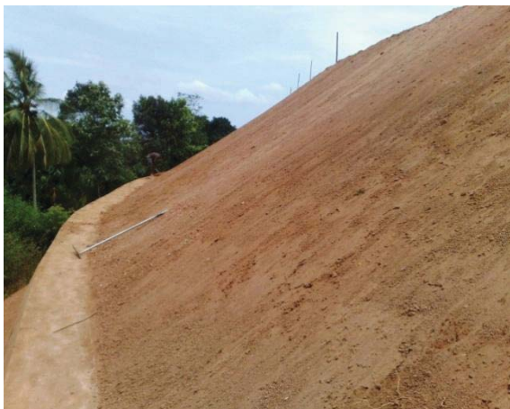
Fig. 3 Prepared slope surface above retaining wall.
