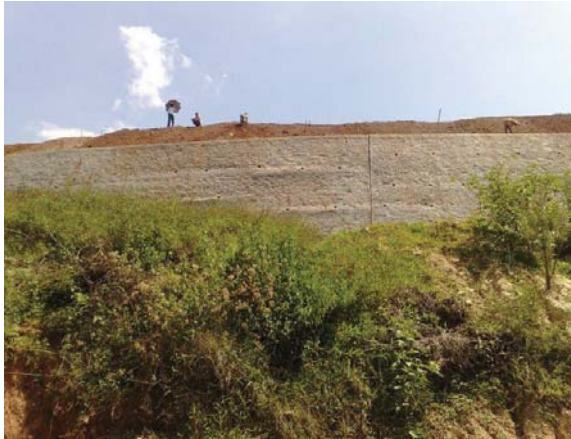
Fig. 2 Construction of fill over the retaining wall is in progress
