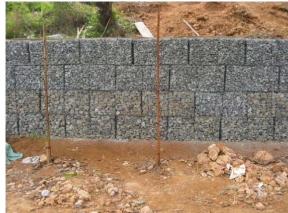
Fig. 10 Front view of the completed gabion facing retaining wall
