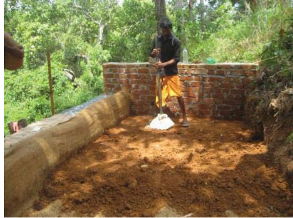
Fig. 9 Compaction of the backfill
