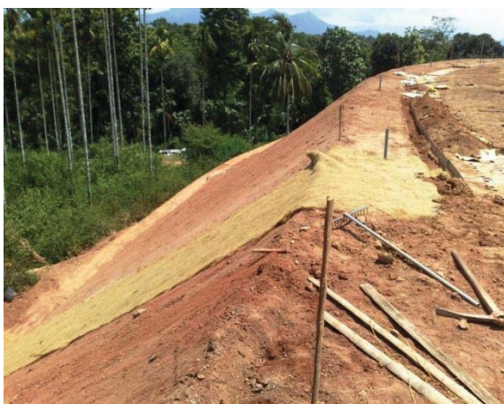
Fig. 4 Laying and fixing of the coir erosion control blanket
