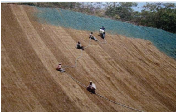
Fig. 11 Hydro seeding over CCM mesh matting.
