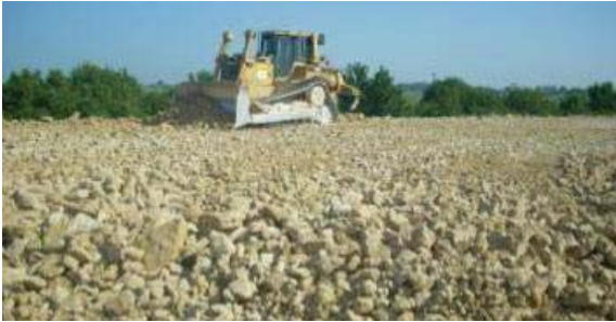
Fig. 16 Leveling with bulldozer on the embankments
