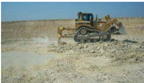
Fig. 11 Rock breaking at the base of the pond
