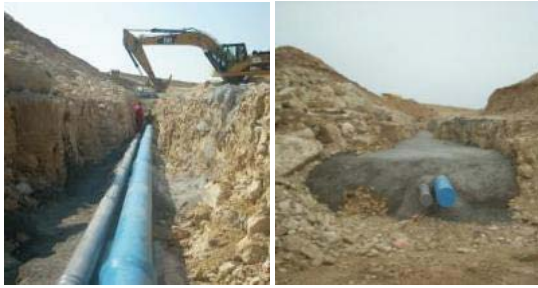
Fig. 23 Outlet and water drainage pipes through the embankment
