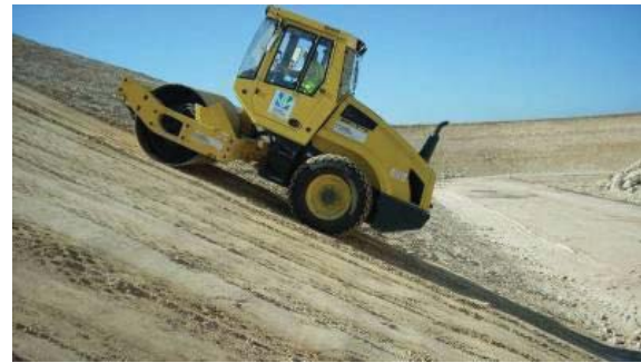
Fig. 20 Final compaction
