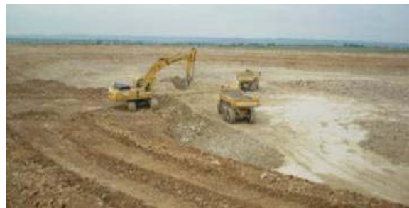
Fig. 14 Excavation of the base of the pond and truck loading
