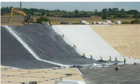
Fig. 31 Unfolding of EPDM geomembrane
