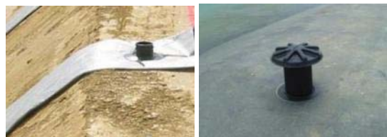
Fig. 28 Gas vent at the top of the embankment
