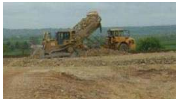
Fig. 15 Unloading of excavated ground on the embankments
