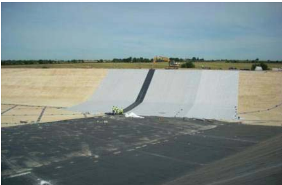
Fig. 30 Unrolling of EPDM geomembrane
