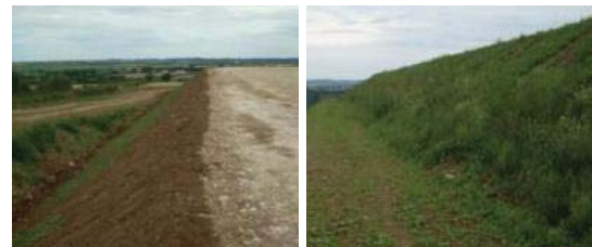
Fig. 22 External embankment (before and after seeding)
