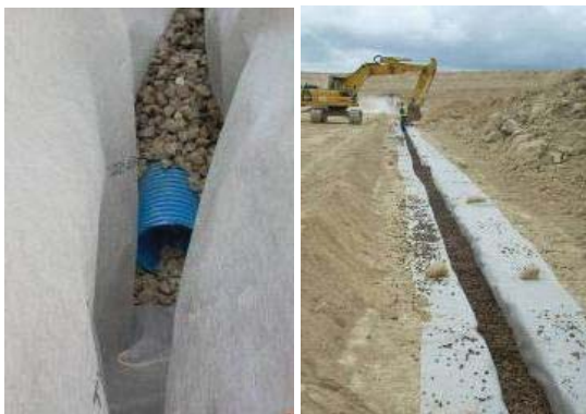
Fig. 25 Water drainage ditch
