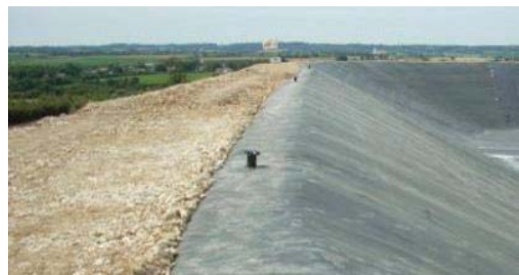
Fig. 35 Anchor trench after back filling
