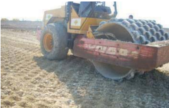
Fig. 16 Compaction of the embankments with chevron tamping wheels compactor
