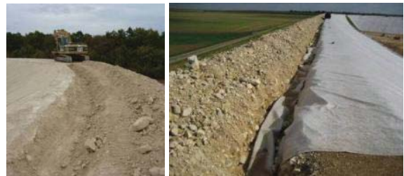
Fig. 34 Anchor trench with geotextile
