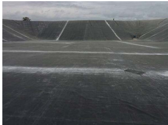
Fig. 33 Installed EPDM geomembrane
