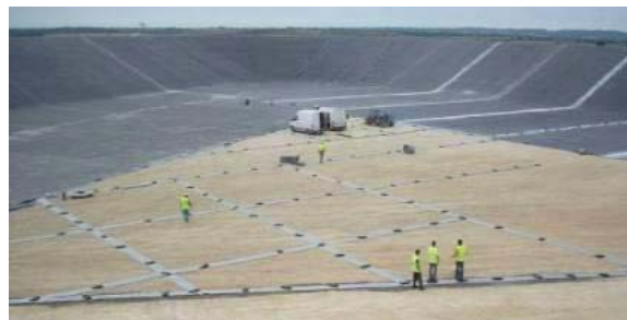
Fig. 27 Gas drainage with geocomposite
