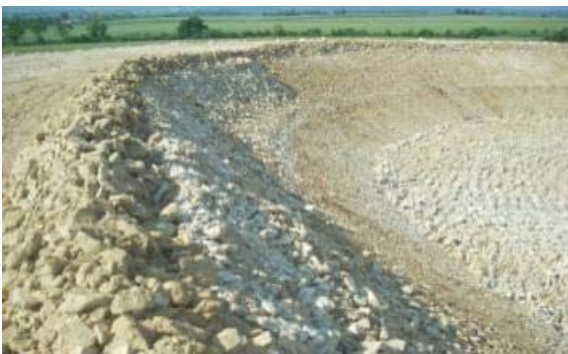
Fig. 18 Embankment before final finishing
