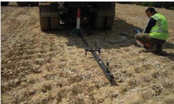
Fig. 17 Measurement of the degree of compaction
