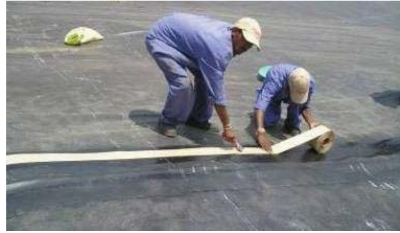
Fig. 32 Seaming of EPDM geomembrane
