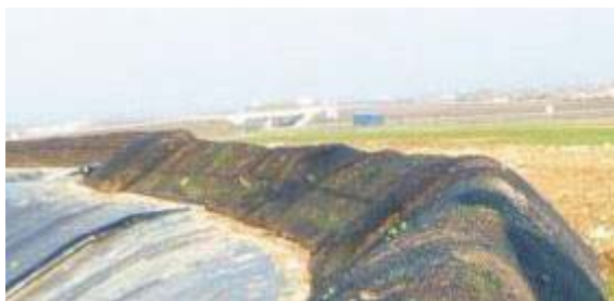
Fig. 38 Waves protection
