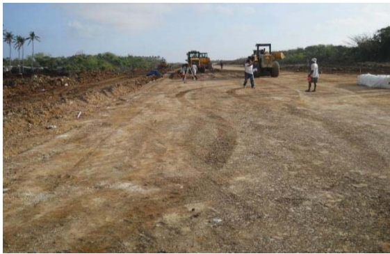
Fig. 8 Compaction of existing platform at minimum 95% density requirement.
