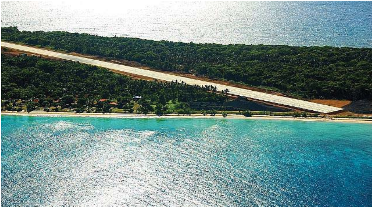
Fig. 13 Constructed runway with MacCell™-reinforced subgrade. (Photo courtesy of Alphaland Corporation.)
