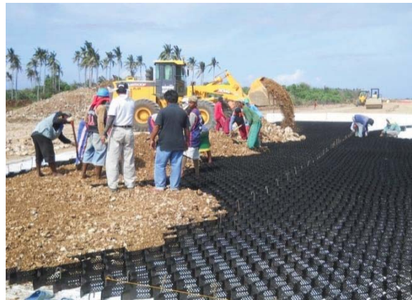
Fig. 12 Backfilling commences soon after enough panels of MacCell™ are laid.
