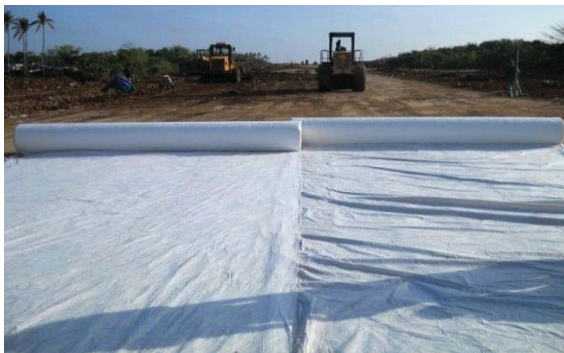
Fig. 9 Laying of geotextile at the prepared base prior to MacCell™ geocells.
