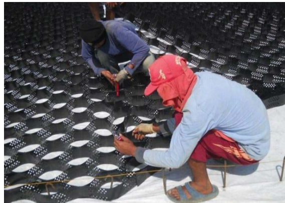
Fig. 11 Connecting ends or sides of MacCell™ panels with handheld equipment.
