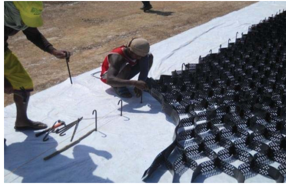
Fig. 10 Installation of guide pins.
