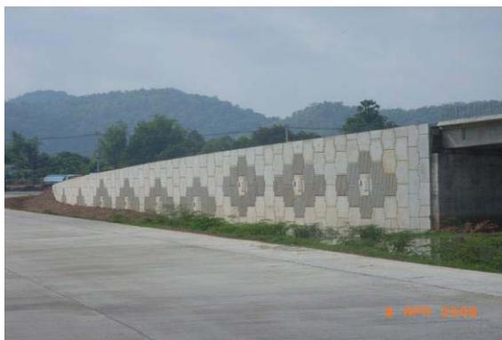
Fig. 3 Application of BRE wall for highway structure in Suraburee Interchange project.
