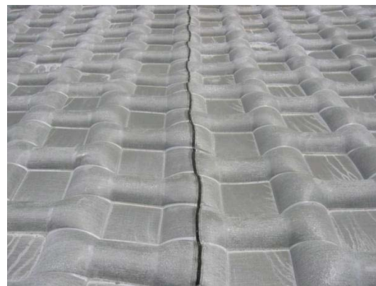
Fig. 4 Industrial zipper connection after filling
