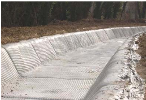
Fig. 13 Irrigation channel with a geosynthetic concrete mattress as sealing system.
