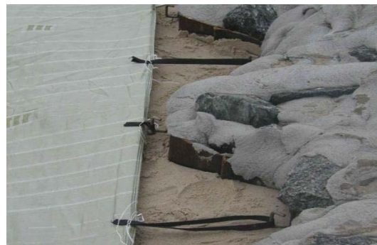
Fig. 17 Connection with sheet pile (unfilled mattress)
