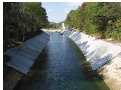
Fig. 15 Sealing of a power plant intake channel with the Standard mattress.
