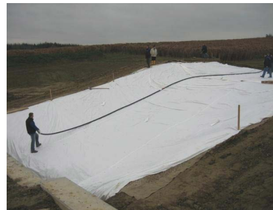
Fig. 7 Installation – laying out mattress.
