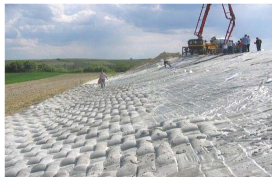
Fig. 11 Overflow section during installation of mattress (2008).
