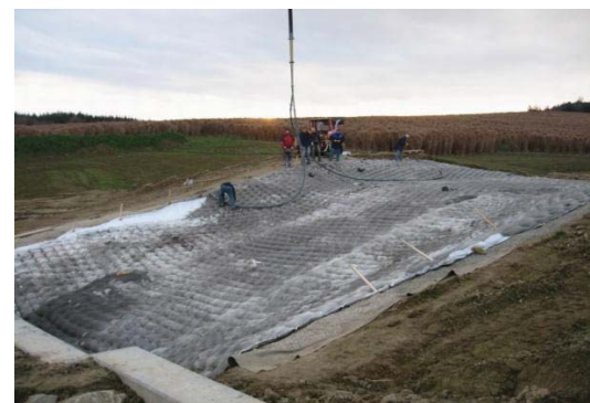
Fig. 8 Installation – filling mattress.
