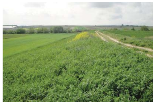
Fig. 12 Overflow section (see Fig. 10) two years after mattress installation (2010).
