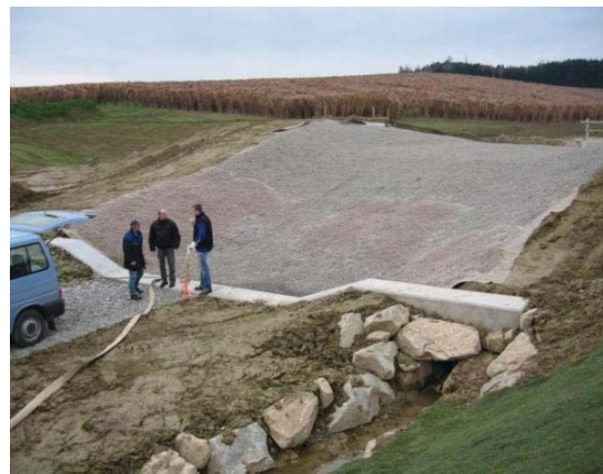
Fig. 6 Installation – preparing under layer.
