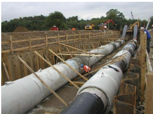
Fig. 19 Concrete mattress as negative buoyancy for an inverted siphon.
