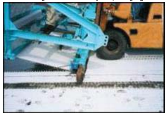
Fig. C3 Specially fabricated brushes prevent wrinkles on the fabric.
