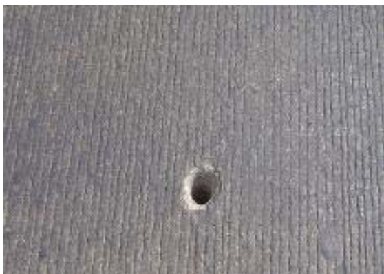
Fig. E1 Sealing of base course with cement grout.
