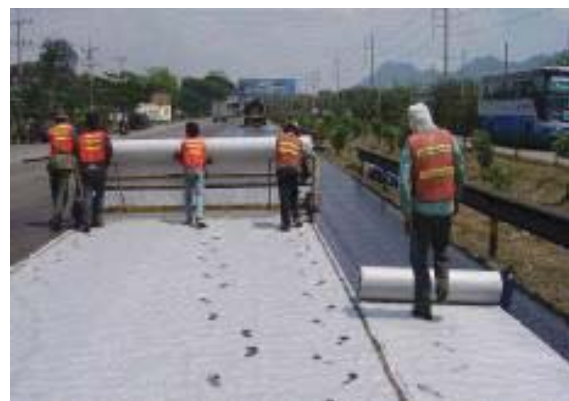
Fig. E3 Installation of paving fabric.
