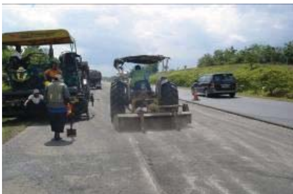
Fig. D1 Milling of old pavement.
