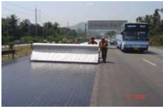
Fig. 2 Laying paving fabrics.
