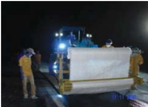
Fig. A4 Installation of PGM-G50/50 paving fabric onto tack coat.
