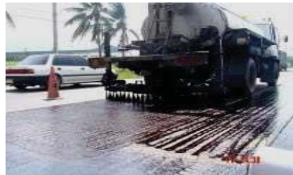
Fig. 1 Spraying of bitumen.
