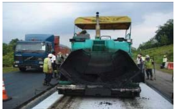
Fig. D4 Tipping of asphalt concrete
