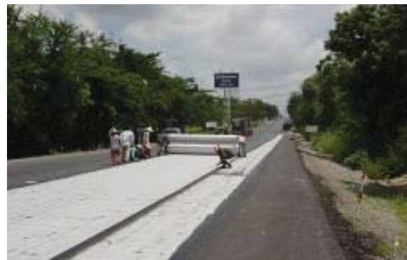
Fig. E4 Butt joint along the length of the paving fabric.
