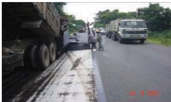
Fig. 3 Overlaying with asphalt.
