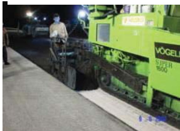
Fig. A6 Overview of asphalt concrete being discharge from track loader.
