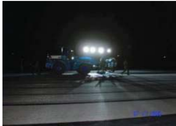
Fig. A5 Overview of installed paving fabrics.
