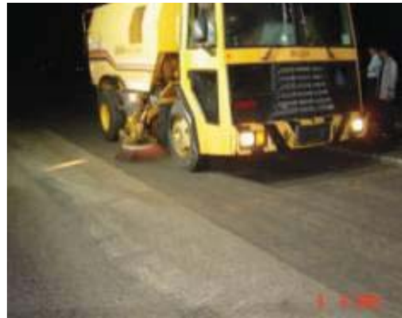
Fig. A2 Cleaning of dust from milled area.
