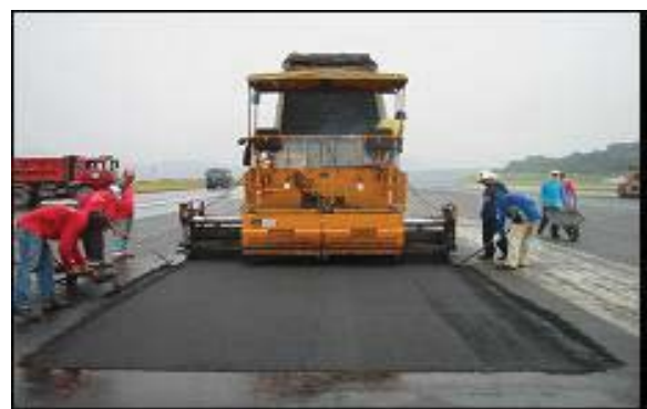
Fig. B4 Tipping of asphalt concrete and its uniform spreading.
