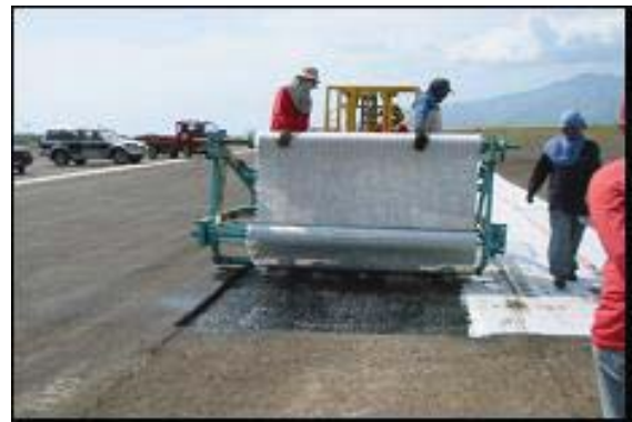
Fig. B3 Installation of PGM-G paving fabric utilizing Polyfelt custom rig.
