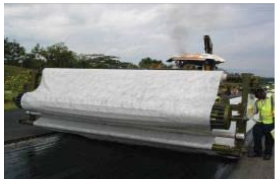
Fig. D3 Installation of PGM 14 paving fabric.
