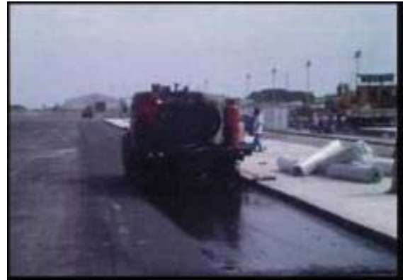
Fig. C1 Tanker with controlled spray bar for initial pure bitumen application.
