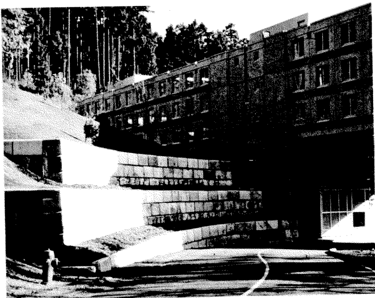
Fig. 2 Tiered geosynthetic reinforced soil segmental retaining wall with 0.75m x 0.75m x 1.5m solid concrete units (Bowden 1991).
