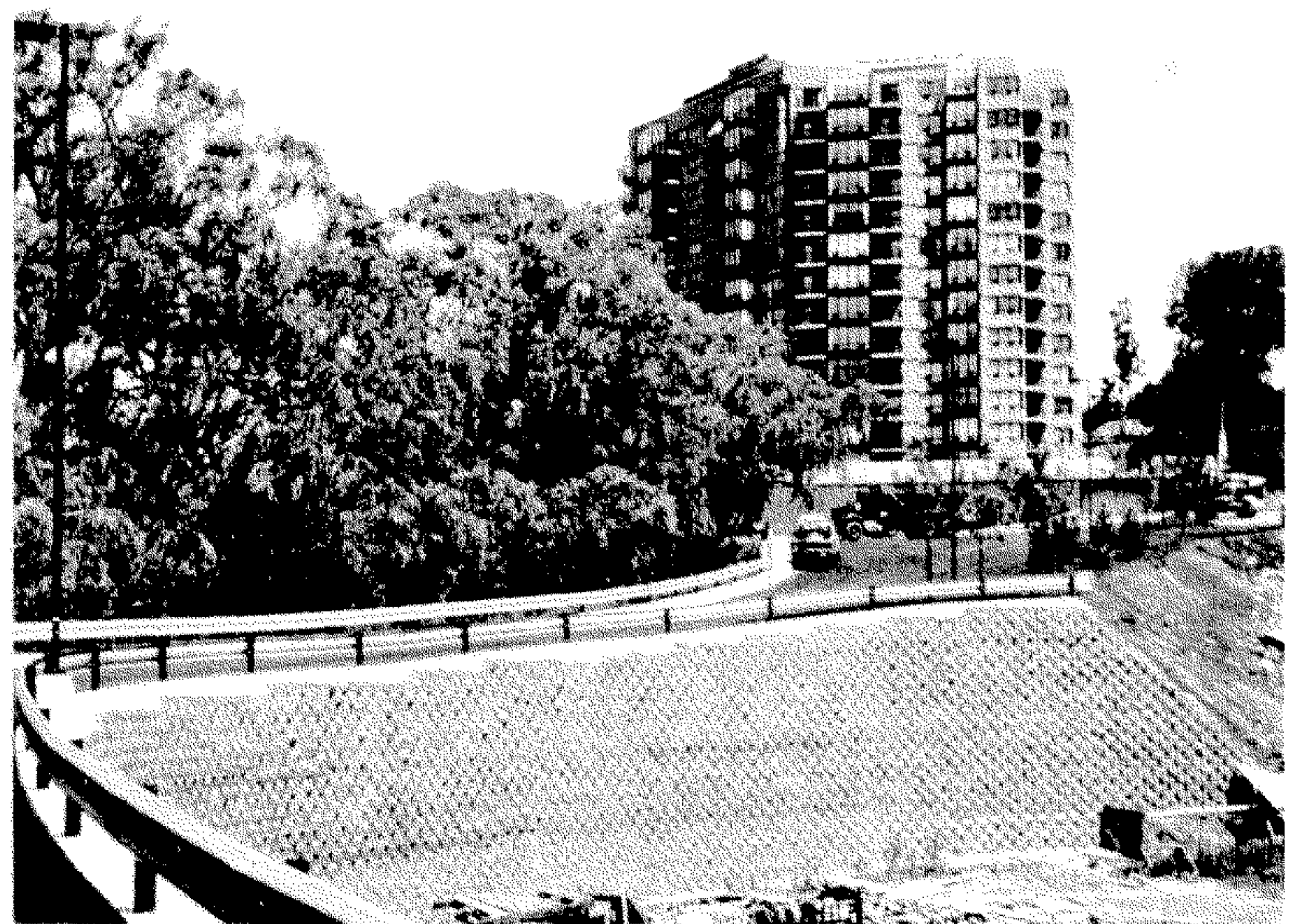
Fig. 1 First major geosynthetic reinforced soil segmental retaining wall structure built in Canada (7 m height) (Crowe et al. 1989).
