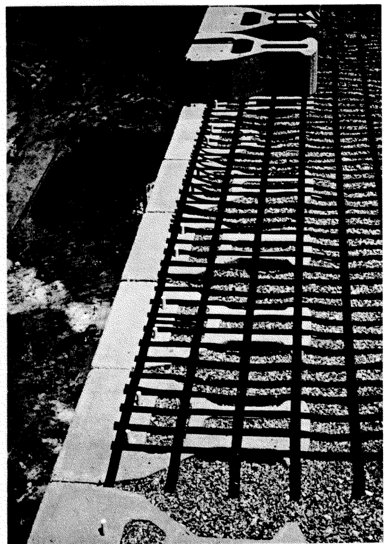
Fig. 26 Facing detail (California wall).
