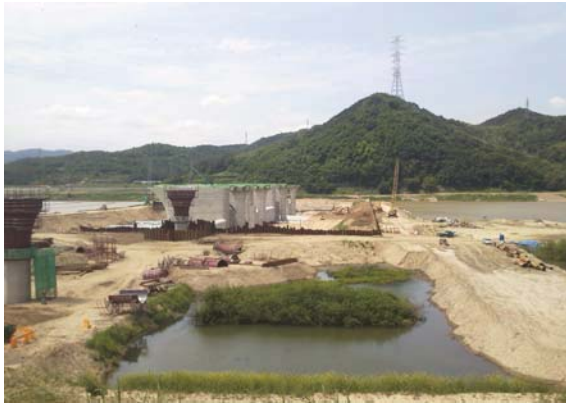
Fig. 15 Completed first phase geotextile tube cofferdam
