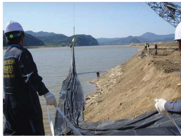
Fig. 13 Laying of geotextile tube
