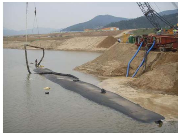
Fig. 14 Pumping of geotextile tube
