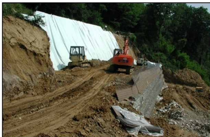
Fig. 3. Example of drainage at the back of the RSS and of internal drainage system
