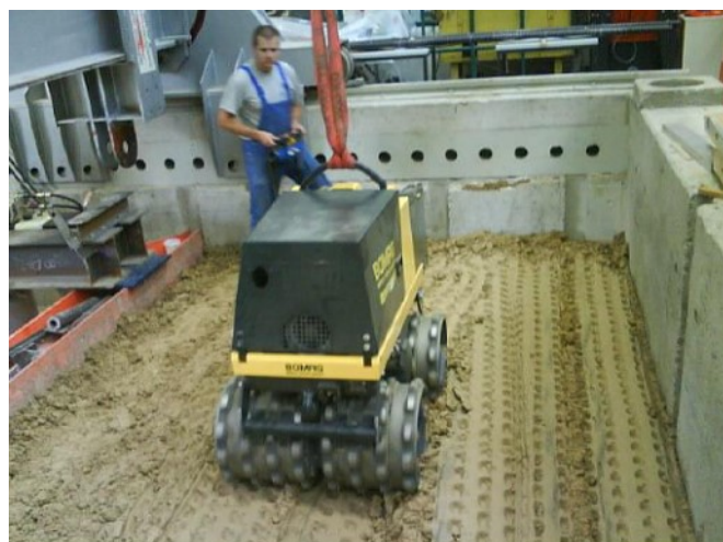
Figure 9. Subsoil installation for the large-scale tests
