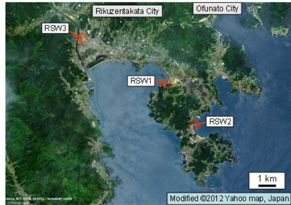
Figure 4. Reinforced soil walls in Rikuzentakata City (Kuвано et al., 2012, 2014).
