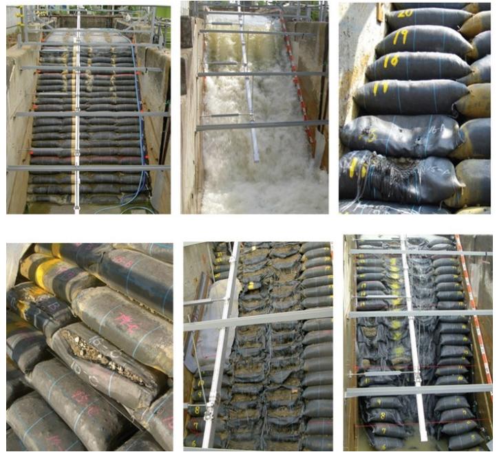
Figure 27. Eroded surface of Soil bags
