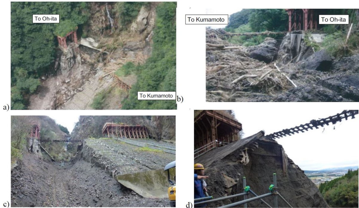
Figure 18. a) Aerial photograph; and b) a close view from upstream (a & b: immediately after the 2012 heavy rainfall, by the courtesy of JR Kyushu); and c) a view from the downstream; and d) exposed cross-section of geosynthetic-reinforced section (c & d: taken 26 November 2012). Site 2 of Ho-hi Line, JR Kyushu (Tatsuoka et al., 2007).
