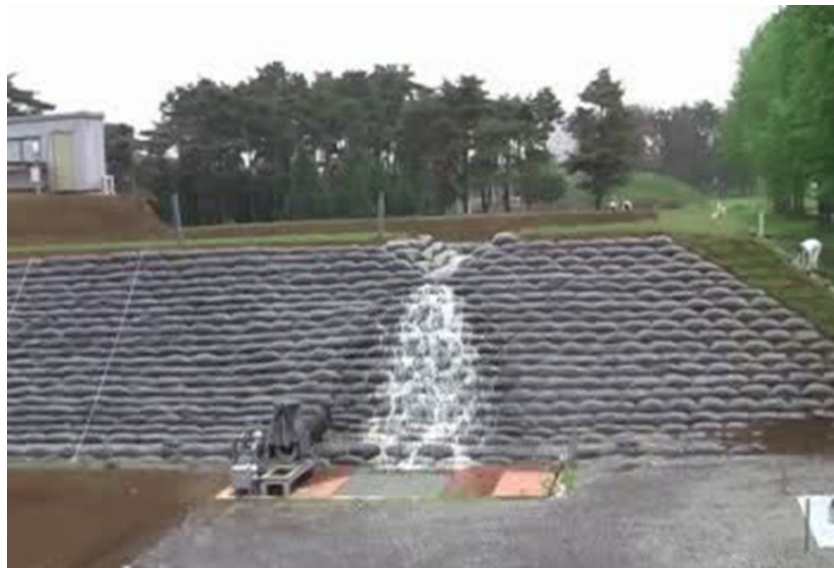
Figure 29. Overflow test of spillway of the full-scale field model earth-fill dam.
