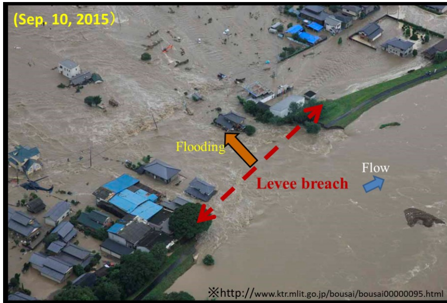
Figure 38. Levee breach in Kinugawa River was caused by extreme flood due to typhoon No. 18.
