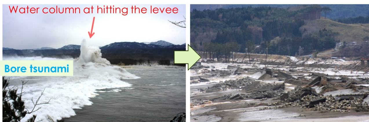
Figure 30. Tsunami and damage of coastal dike at Tofugaura in Iwate Prefecture.
