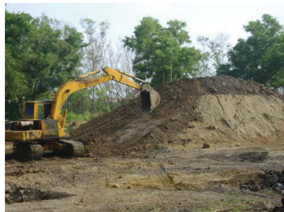
Fig. 4 The construction of embankment slope (1V:1.5H) for monitoring
