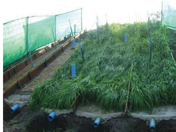
Fig. 9 The embankment at East side
