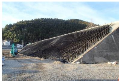
(b) Arranging geo-cell layers
