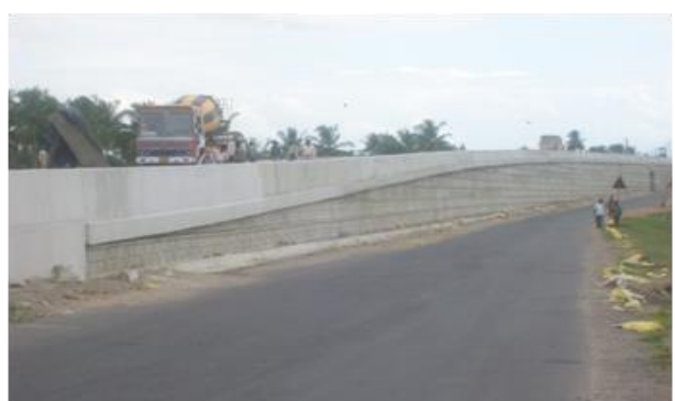
CH: 111+860- Pedestrian Underpass
