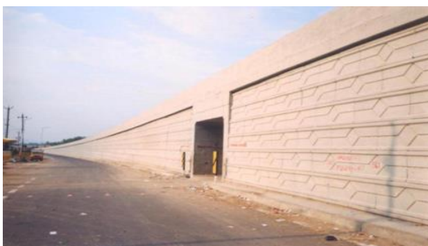
CH: 108+440- Pedestrian Underpass
