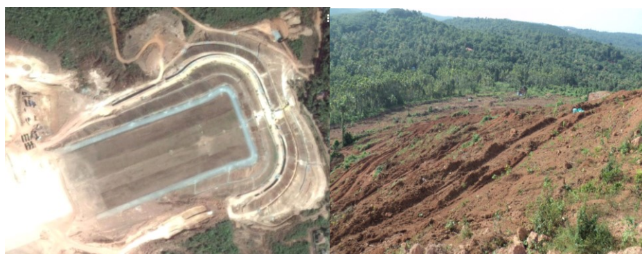
Figure 2. (a) Google earth image of Runway End Safety Area (b) Project site before construction
