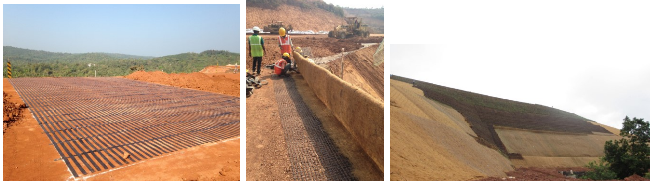
Figure 5. (a) Geogrid Laying (b) Welded mesh fascia with coir mat (c) Erosion control measures
