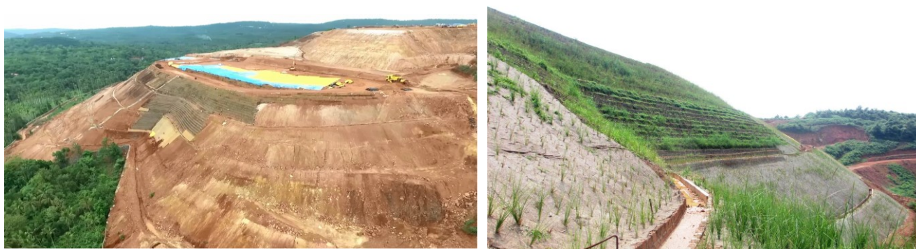
Figure 6. (a) Overall view of the slope (b) Reinforced soil slope
