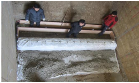
(a) Compact soil in Geotube (b) Compact soil in wire mesh with Geotube Figure 2 Keystone installation procedures of proposed method
