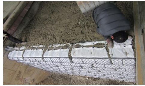
(a) Compact soil in Geotube (b) Compact soil in wire mesh with Geotube Figure 2 Keystone installation procedures of proposed method
