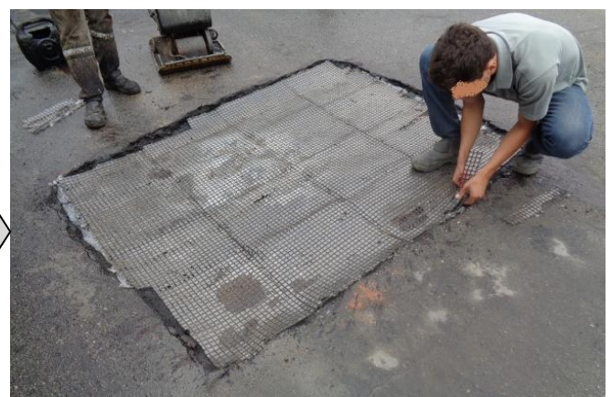
Carbon fiber grid positioned
