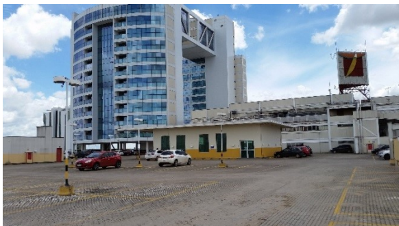
Figure 5. View of the outer parking lot from the top floor.
