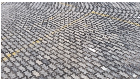
Figure 6. View of the interlocking floor in the outer parking lot of the upper floor.
