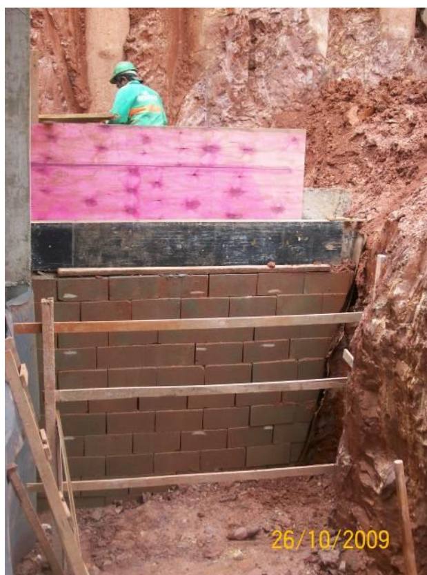
Figure 21. View of the wooden jig mounted in front of the wall.
