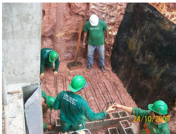
Figure 17. Application of the arching tapes in the second layer.
