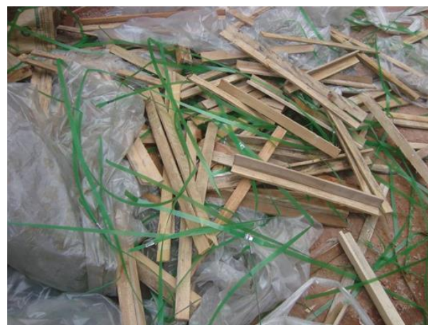
Figure 3. Discarded tapes in the works of Águas Claras, Federal District (DF).
