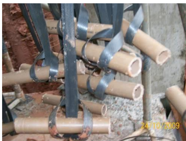
Figure 16. Views of the mooring of PVC pipes.
