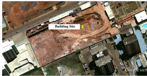
Figure 8. View of the execution site of the wall.
