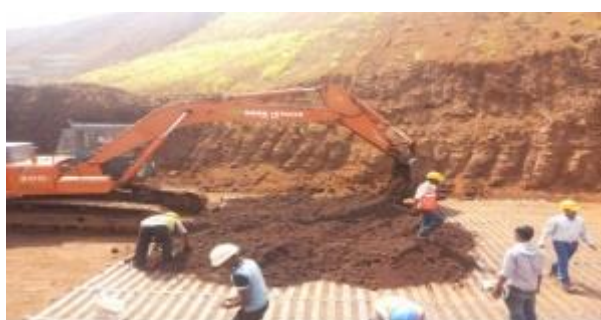
Figure 8. Backfilling Process on going
