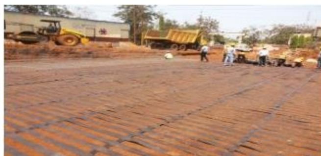
Figure 6. Laying of ParaLink as soil reinforcement
