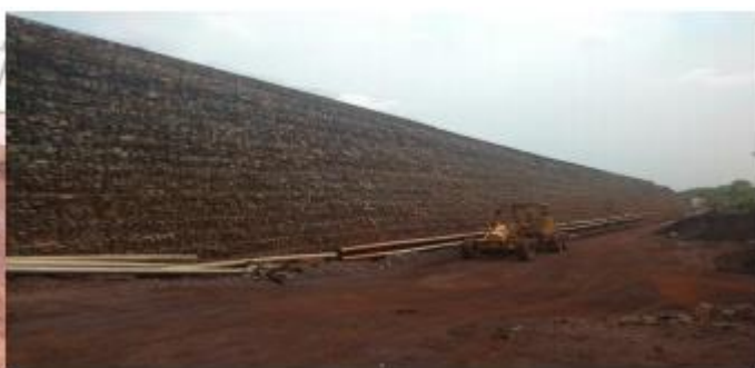
Figure 11. Final stage of Terramesh System Unit
