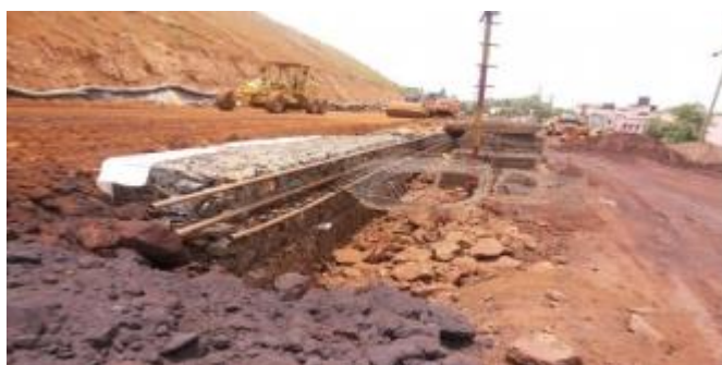
Figure 10. Execution of construction of second layer
