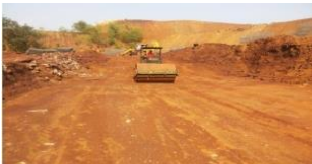
Figure 5. Construction of foundation and compaction
