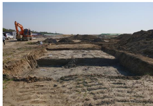
(b) Ground excavation
