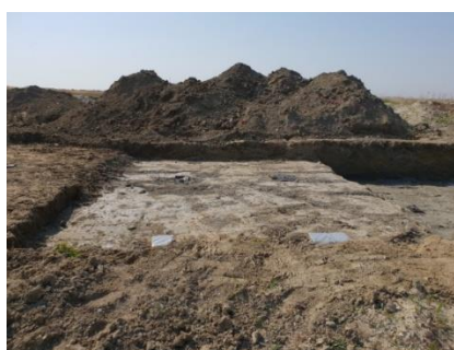
(c) Buried detecting material (0.25m depth)
