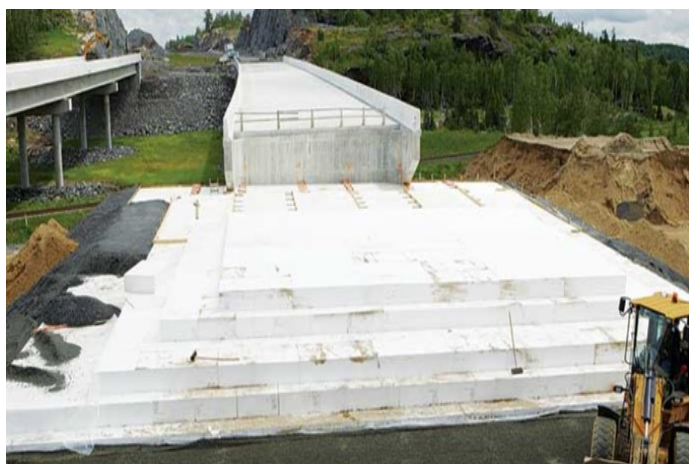
Figure 2. EPS block for embankment
