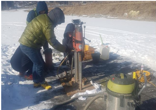
a) Drilling the cavity
