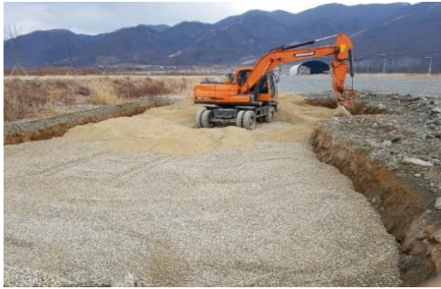
a) Drainage layer and base layer
