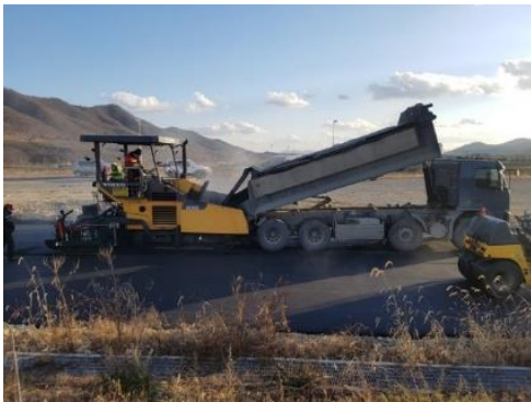
c) Asphalt surface layer
