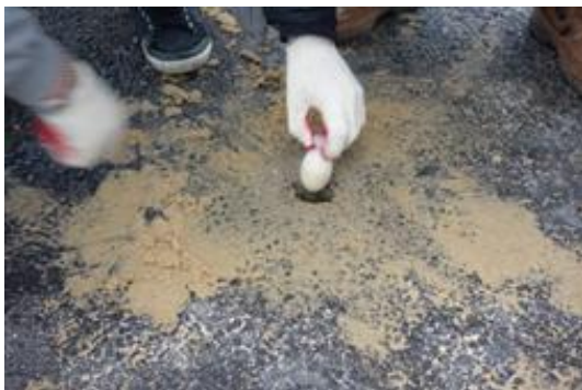
c) Injection of expansive material
