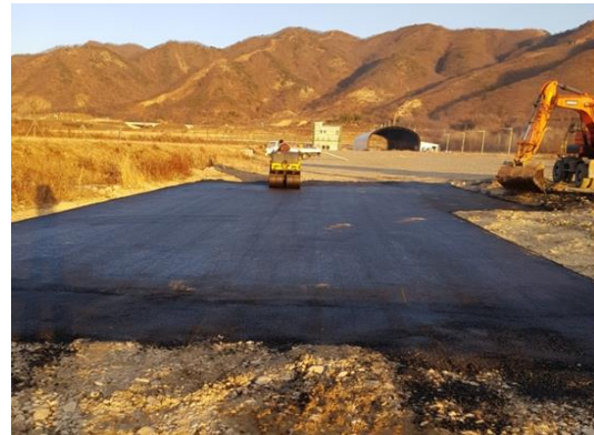
d) Surface layer tamping
