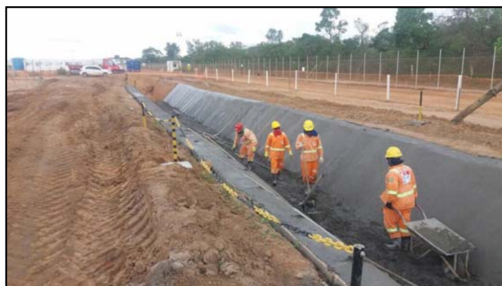
Figure 13. Photovoltaic plant in Bom Jesus da Lapa, BA.
