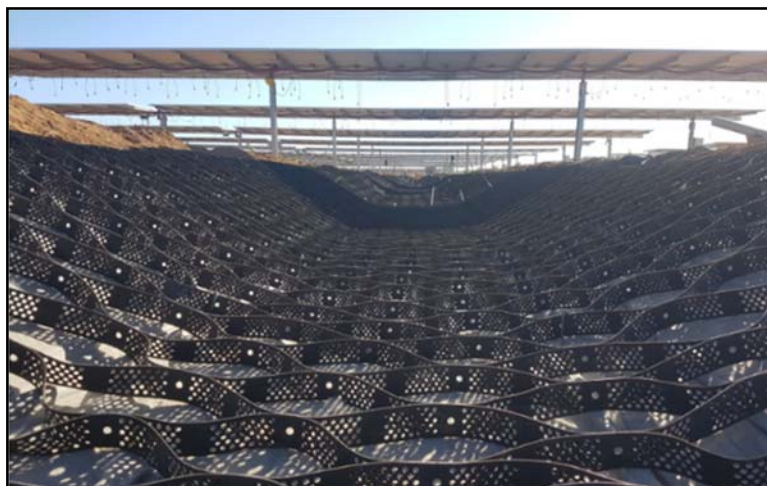
Figure 1. Using HDPE geocells for channels.
