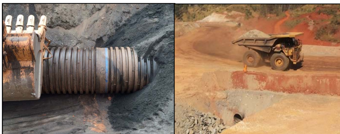
Figure 10. Piping connection and end of work in full operation.
