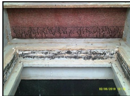
Figure 10. Typical downstream view with sediment-laden discharge
