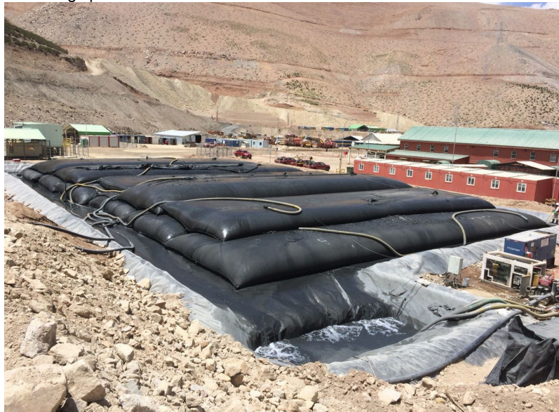
Figure 5. Stack Geotextile tube
