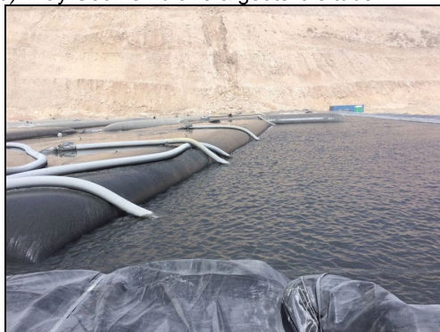
(c) Filling and dewatering
