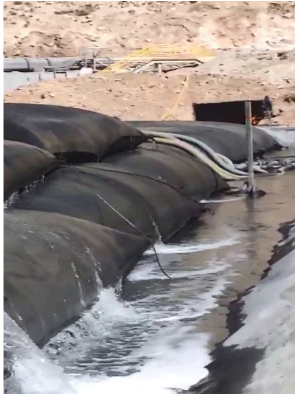
Figure 6. Excellent permeability geotextile tube
