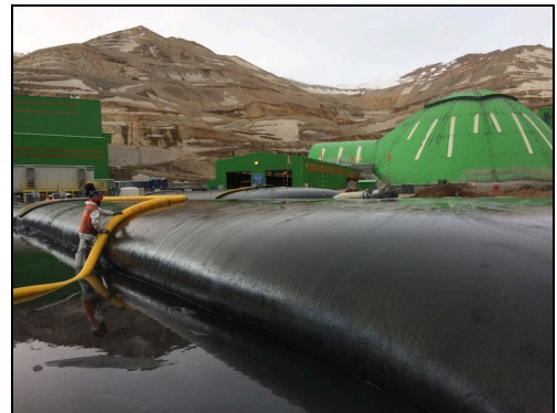
(b) Fill the geotextile tube with tailing slurry
