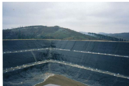
Figure 10. Upstream facing of a dam (Dam Geology. 2011)
