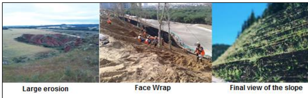
Figure 15. Erosion Control (Geosolutions. 2019)
