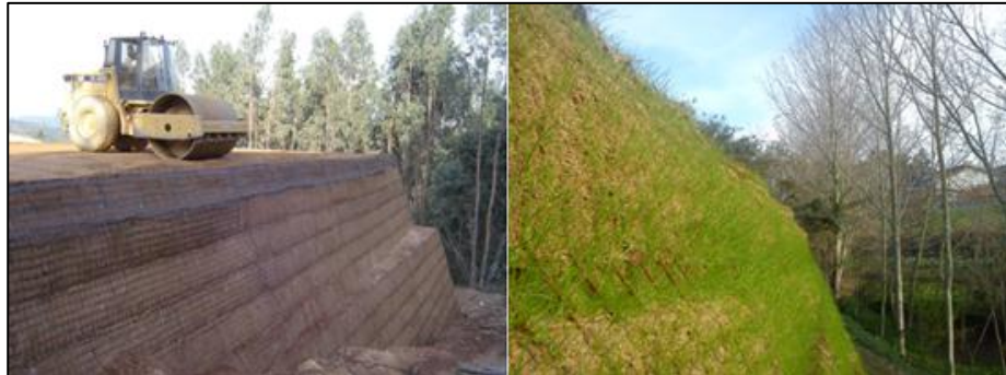
Figure 11. Armed earth retaining wall (ECO SALIX-Ecological Systems of Natural Engineering. 2019)
