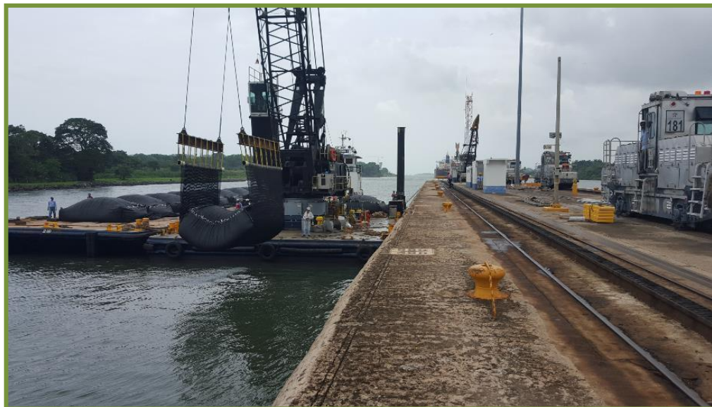
Figure 14 Installing Geobag® Units Along Gatun Locks Dividing Wall
