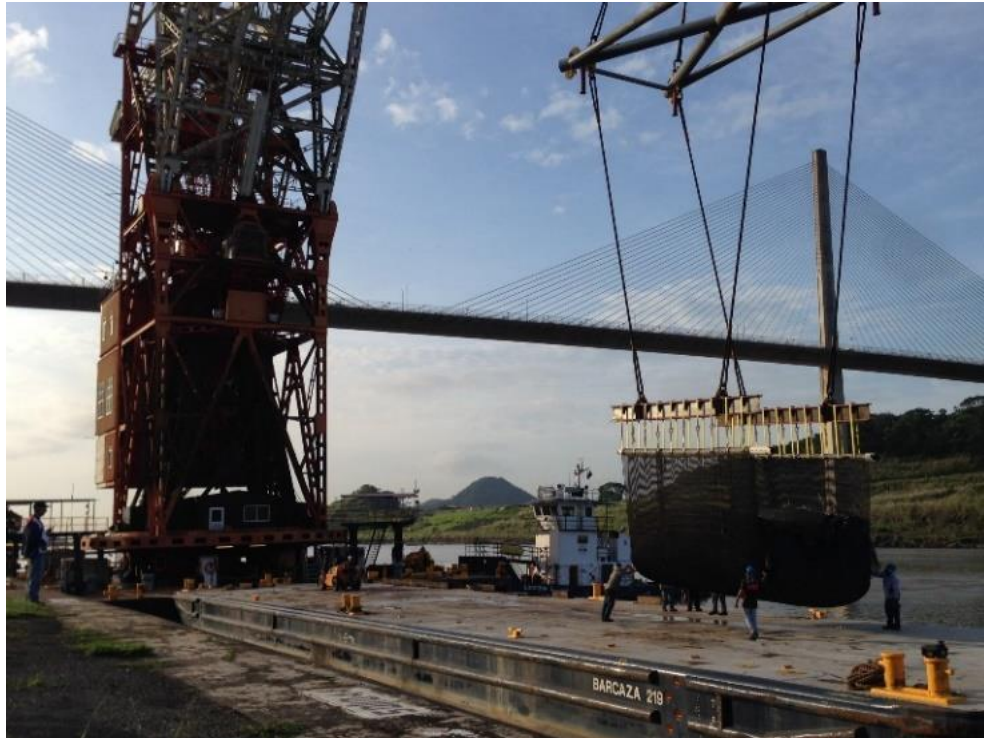
Figure 9 The 300 Ton Crane Placing the 90 Ton Geobag® Containers on Transfer Barge
