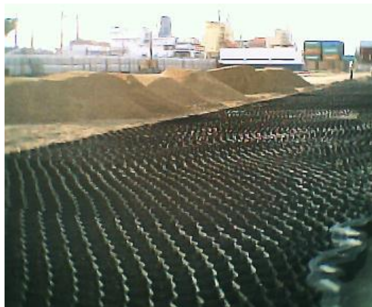
Figure 7: Construction process of Geoweb system (Callao Port).
