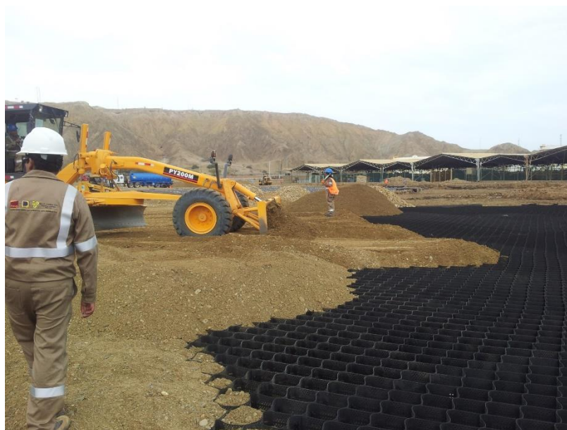
Figure 9: Construction process of Geoweb system (Talara - Piura).
