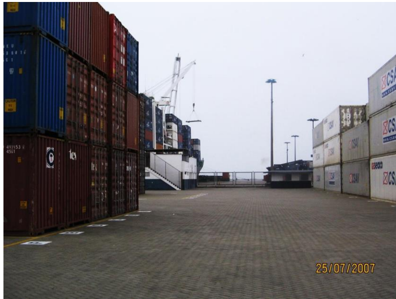
Figure 8: Callao Port -Project finalized.
