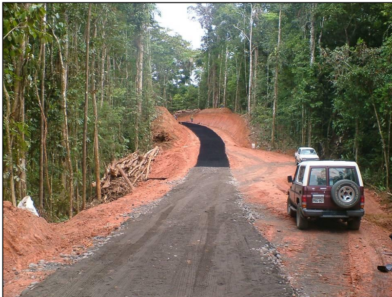
Figure 12: Ecuador Road - Project finalized.
