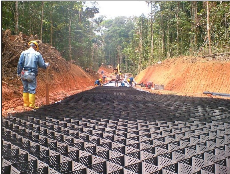
Figure 10: Construction process of Geoweb system (ECUADOR).
