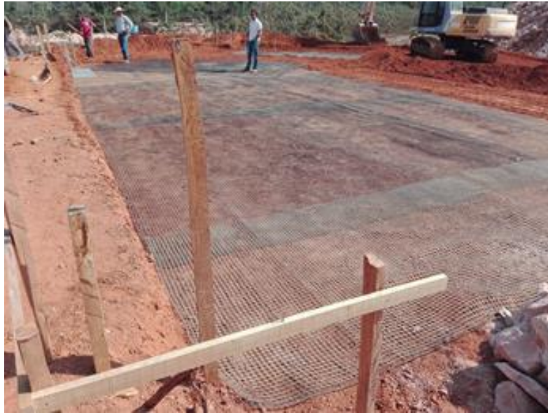
Figure 7. Mounted metal templates for positioning.
