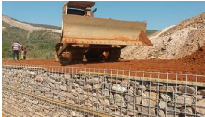
Figure 9. Reinforced soil layers at crusher wall
