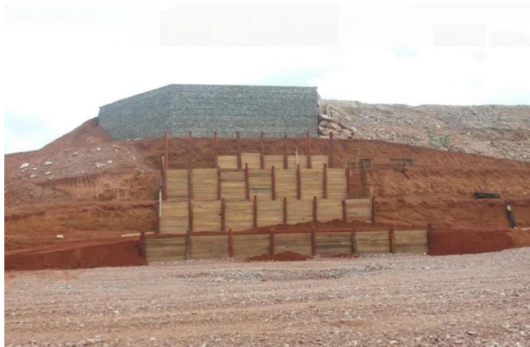
Figure 10. Completed Containment - Quadrate Stone
