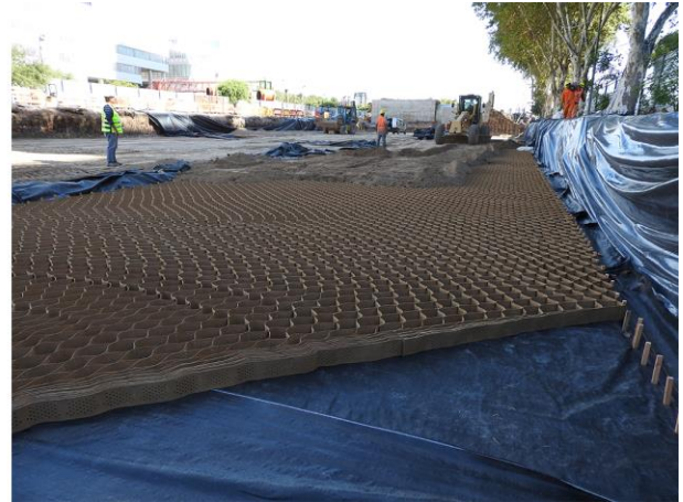
b) Lay down of geotextiles and geocells
