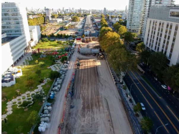
a) Embankment construction area
