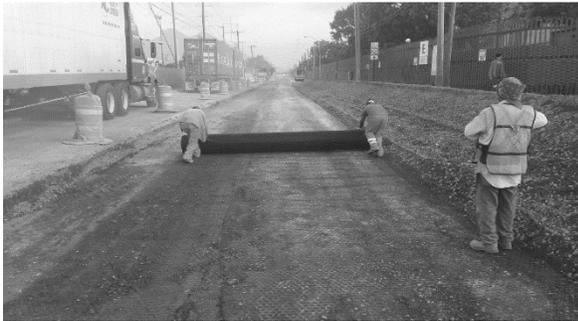
Figura 9. Geomalla multiaxial colocada
