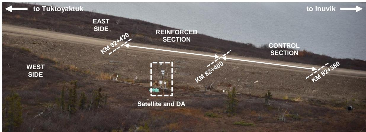
Figure 2. Aerial view of the completed test sections along the highway.
