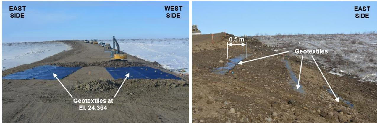
Figure 3. Wicking geotextiles in the reinforced embankment section: (a) installation of wicking geotextile and (b) geotextile overhang for wicking function.
