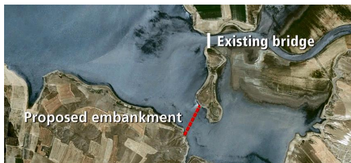
Figure 1. Location of Proposed Embankment.
