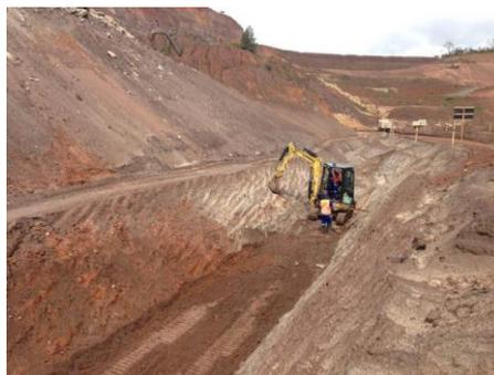
Picture 1 *Excavation of 3m deep channel*
