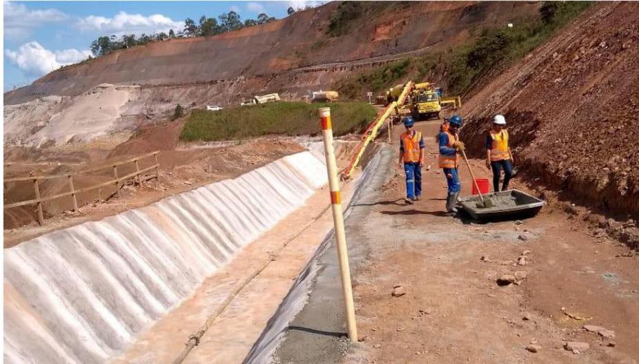
Picture 4 Completed channel and backfilling of anchor trenches using mortar
