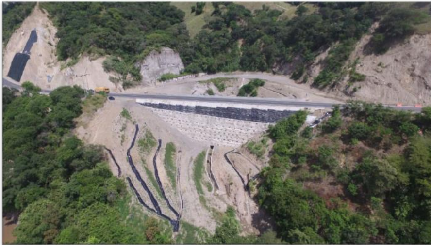
Figure 3 Wall in reinforced ground finished
