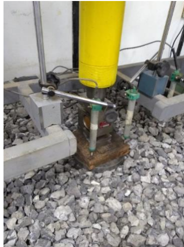
Figure 10. Displacement meter installation
