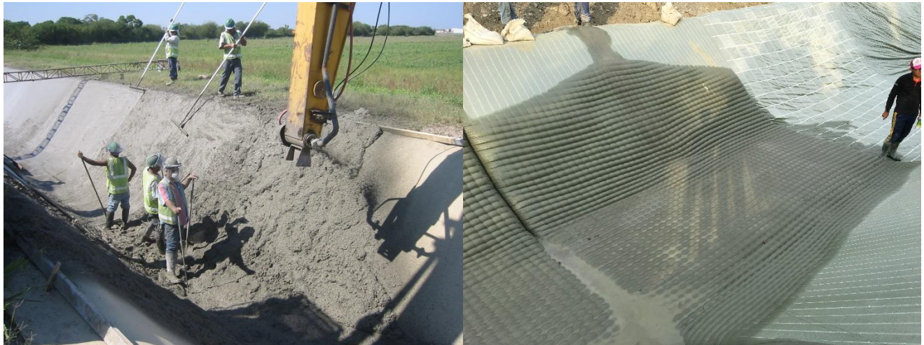
a) Shotcrete application on the membrane composite
